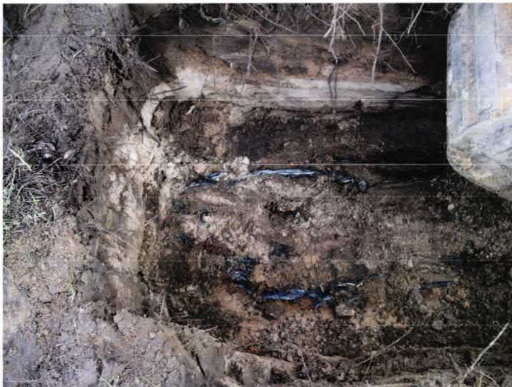
Picture 2: UST 739Bluebell excavation in progress.
